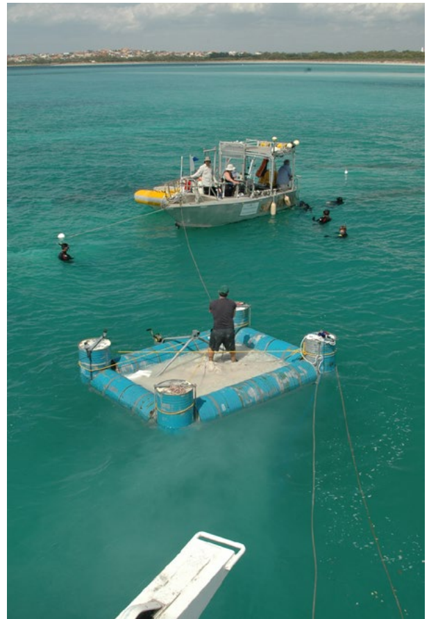
Figure 4. Dumping of sand from the custom-built barge on the James Matthews site (J. Carpenter, Western Australian Museum).
