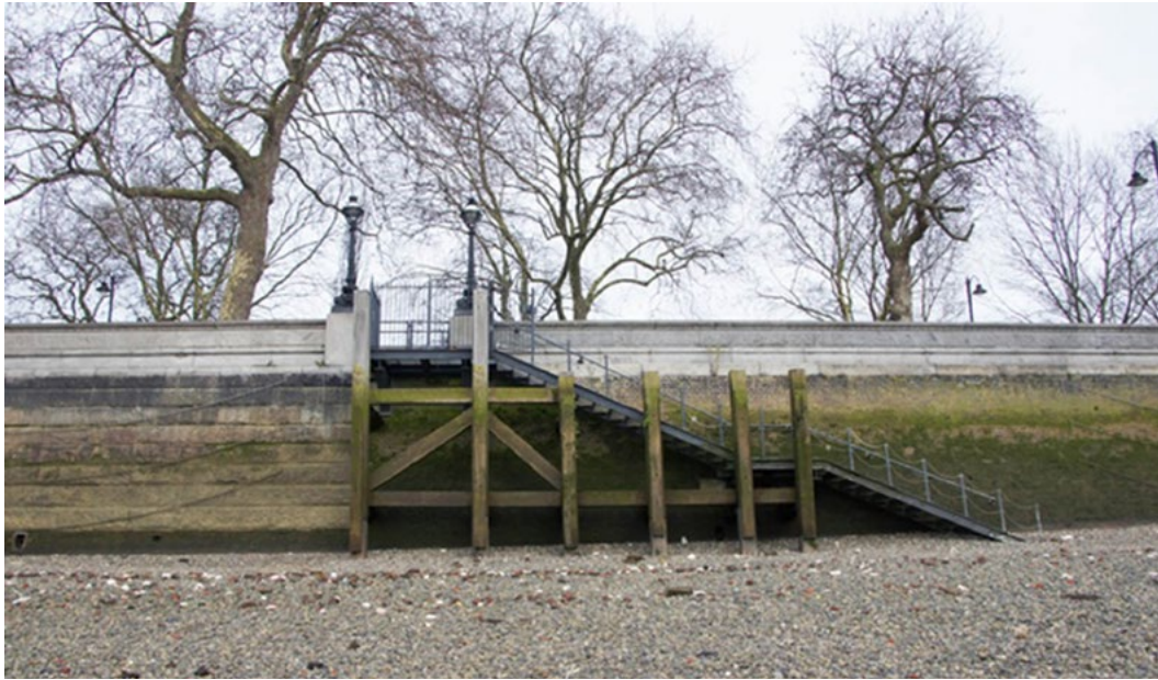
Figure 3. Royal Hospital Stairs, Chelsea. The 1850s embankment is on the right of the river stairs, and is brick built. The 1870s embankment is on the left of the river stairs and is finished with faced granite blocks (Author and Clare Dowling 2016).
